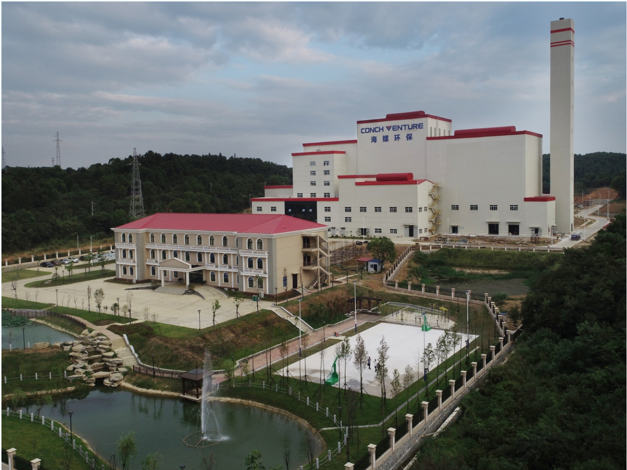
(Pictured: Li county grate furnace power generation project)
