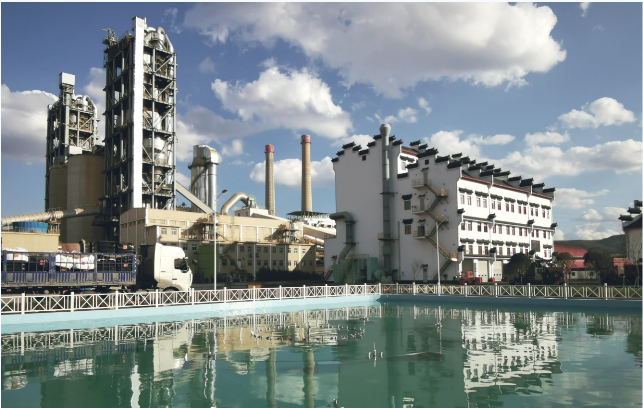
(Pictured: Wenshan treatment of solid and hazardous waste by cement kilns project.)
